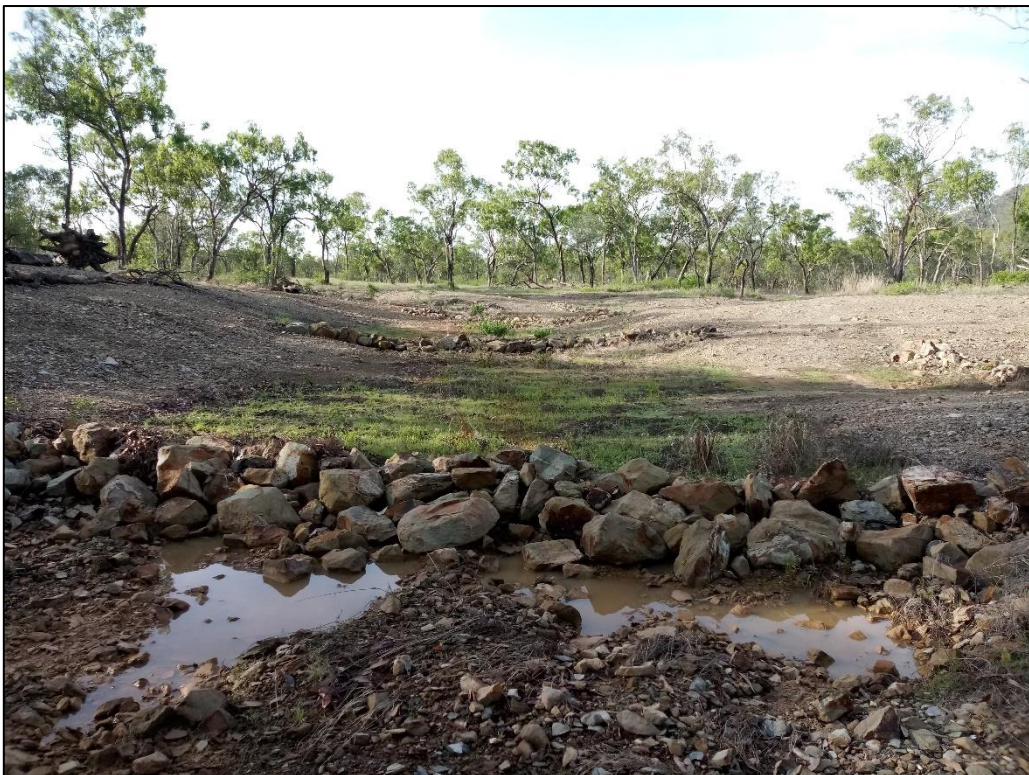
Figure S9C. Looking upstream into remediated gully at same location as Figure SI-9B. Photo taken in on 16/02/2018. Note the check dam has collected coarse sediment and now supports vegetation.
