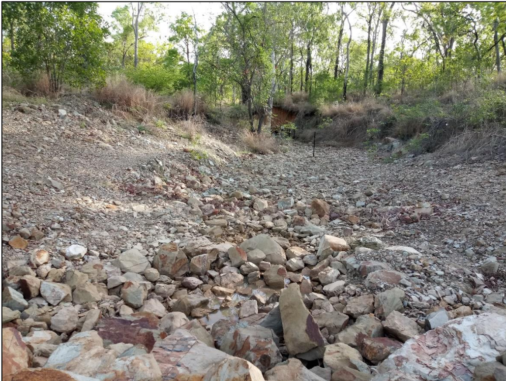
Figure S9B. Looking downstream from at remediated gully head outlet channel. Photo taken in on 16/02/2018. Note the lack of sediment in the channel bed.
