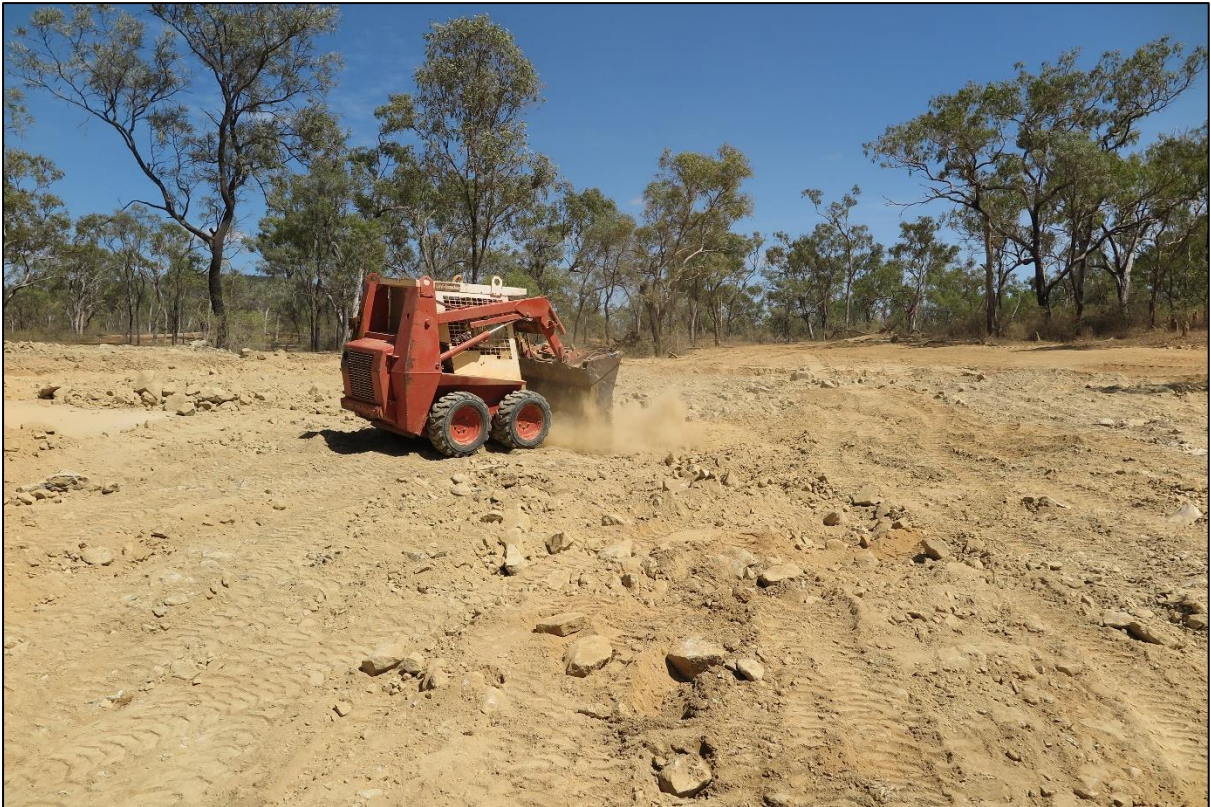
Figure S1F. Rock capping remediated gully.
