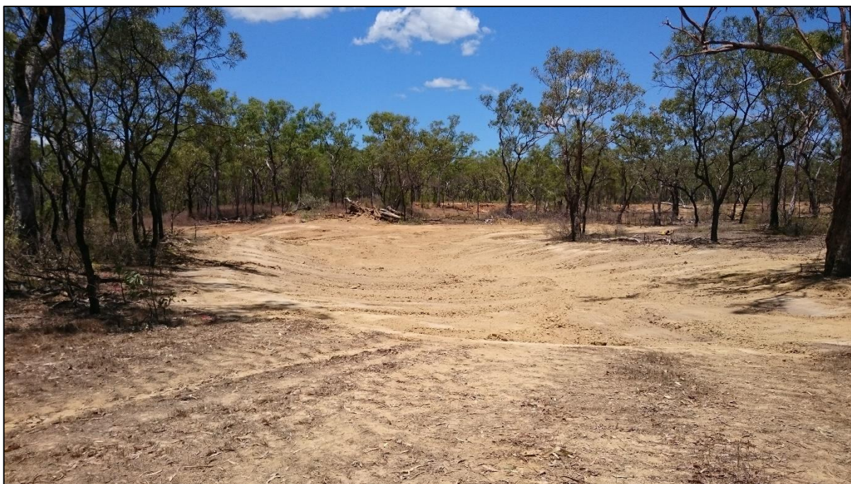
Figure S1C. Finished reshaping of remediated gully.
