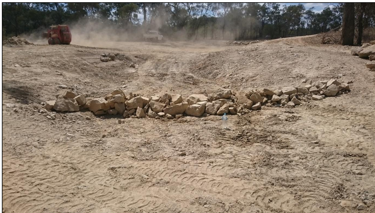
Figure S1G. Remediated gully completed with check dams 2016.
