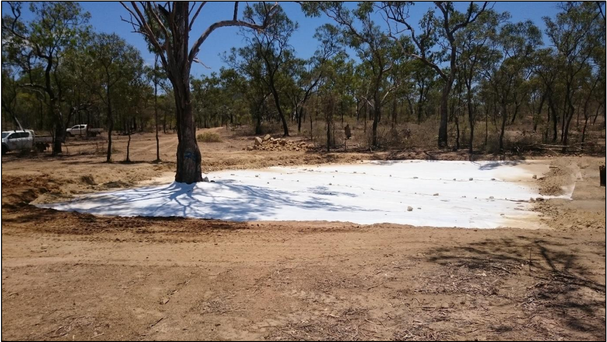
Figure S1E. Geotextile fabric laid over former gully head scarp
