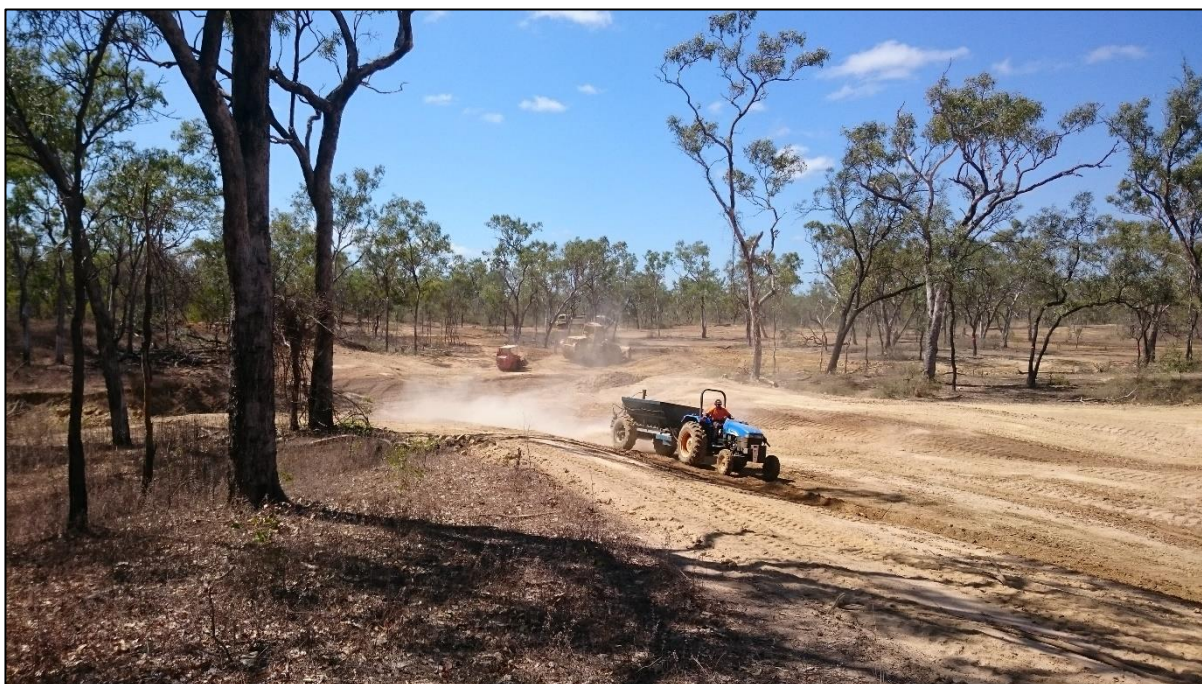
Figure S1D. Spreading gypsum over remediated gully.
