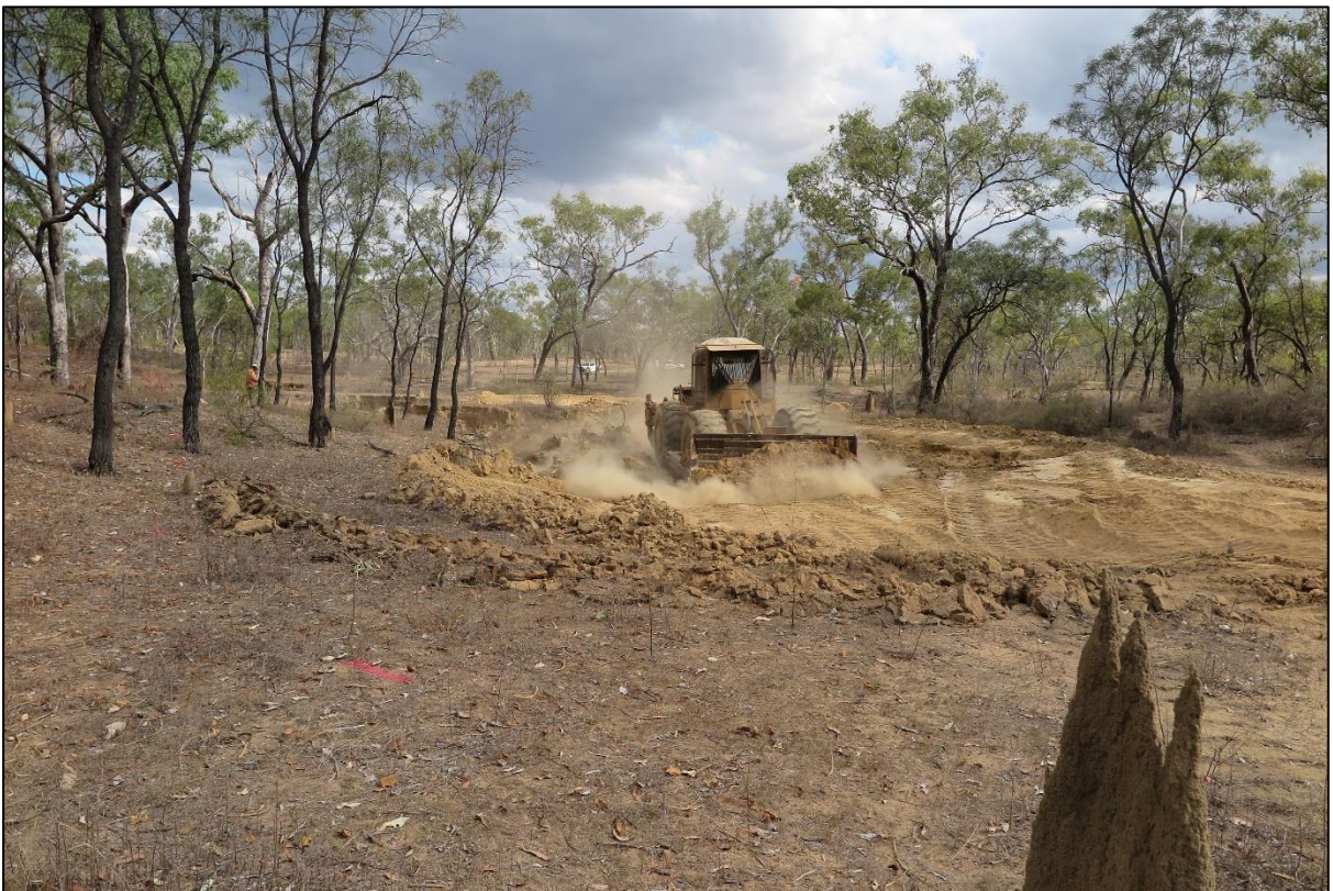
Figure S1B. Reshaping the remediated gully.
