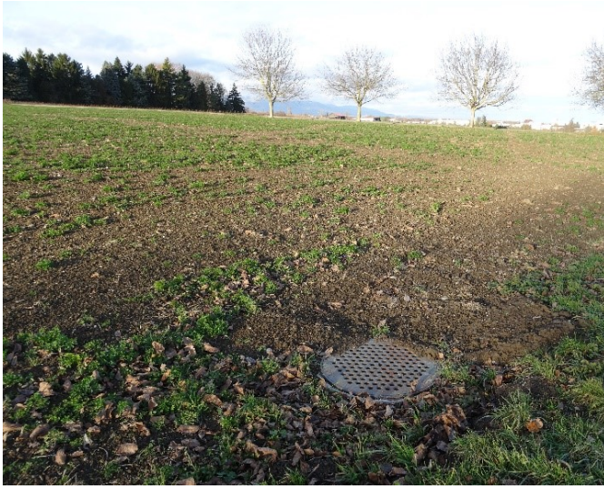
Figure S 5: Storm drainage inlet shaft with a metal grid lid in a field of the study area Meyrin
