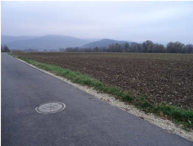
Figure S 8: Maintenance shaft with a concrete lid with a pick hole on a road in the study area Courroux
