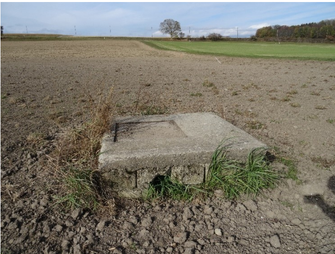
Figure S 10: Tile drainage maintenance shaft in a field in the study area Molondin
