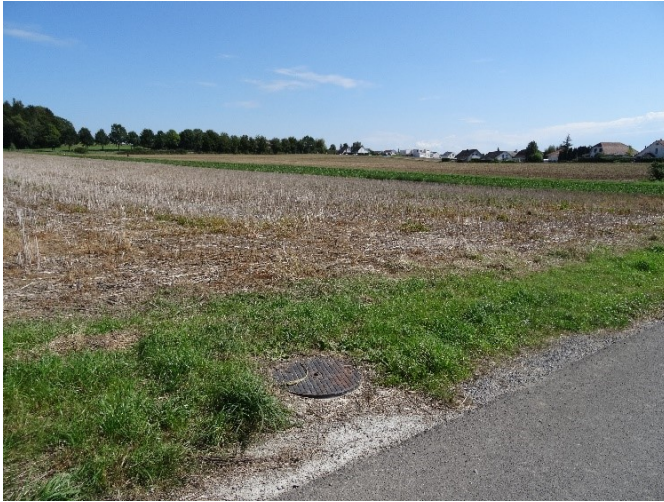
Figure S 7: Maintenance shaft with a metal lid with a pick hole next to a road in the study area Buchs
