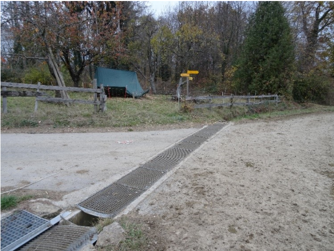
Figure S 11: Channel drain on a road in the study area Clarmont
