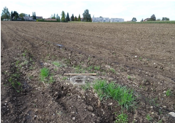
Figure S 6: Storm drainage inlet shaft with a concrete grid lid in a field of the study area Nürens Dorf
