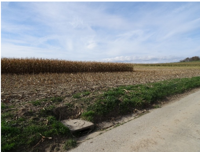
Figure S 3: Lateral concrete storm drainage inlet shaft next to a road in the study area Molondin
