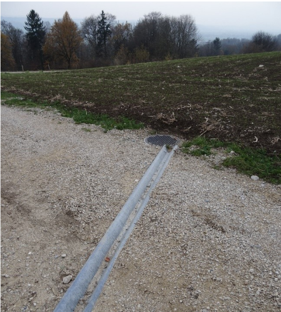
Figure S 12: Channel drain and inlet shaft with a metal grid lid on a road in the study area Lommiswil
