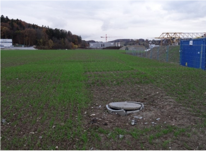
Figure S 9: Damaged tile drainage maintenance shaft in a field in the study area Vufflens-la-Ville
