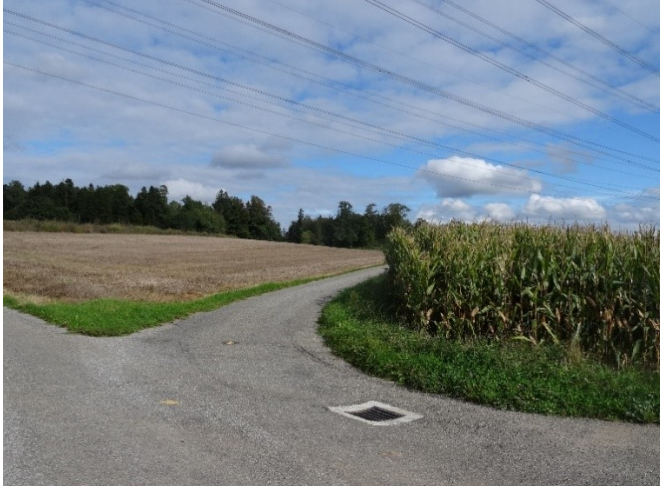
Figure S 2: Storm drainage inlet shaft with a gridded metal lid on a road in the study area Nürendorf
