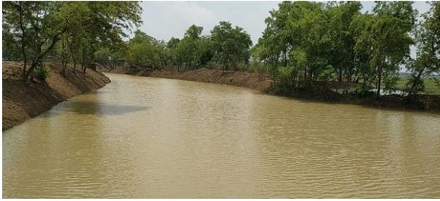
Figure 5. Renovated Ahar–Pyne system in Bihar, India (photo courtesy of Jal Jeevan Hariyali mission, Bihar, India).
