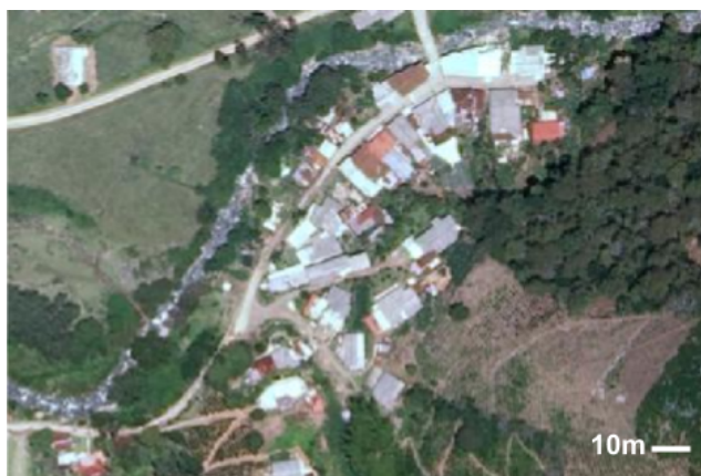
a) Aerial photograph before the event (2012).
