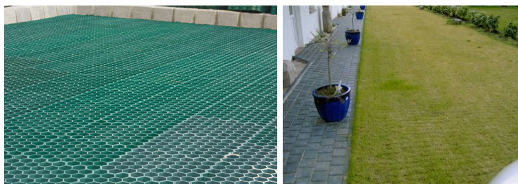
Figure S6: Pavement type D during installation (left) and inside the lawn (right).
