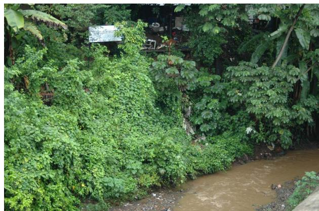
**Fig. 10.** The riverbank protection (live vegetated crib wall and a slope grating) 44 months after cuttings planted and with sedimentation in the lower part.
